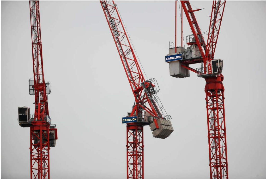
Carillion construction cranes at a building site in London on Sunday. Carillion, a construction company that helped the government run day-to-day operations, filed for bankruptcy.
